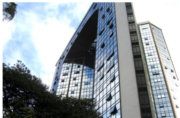
Newly constructed office buildings in Nairobi Central Business District
